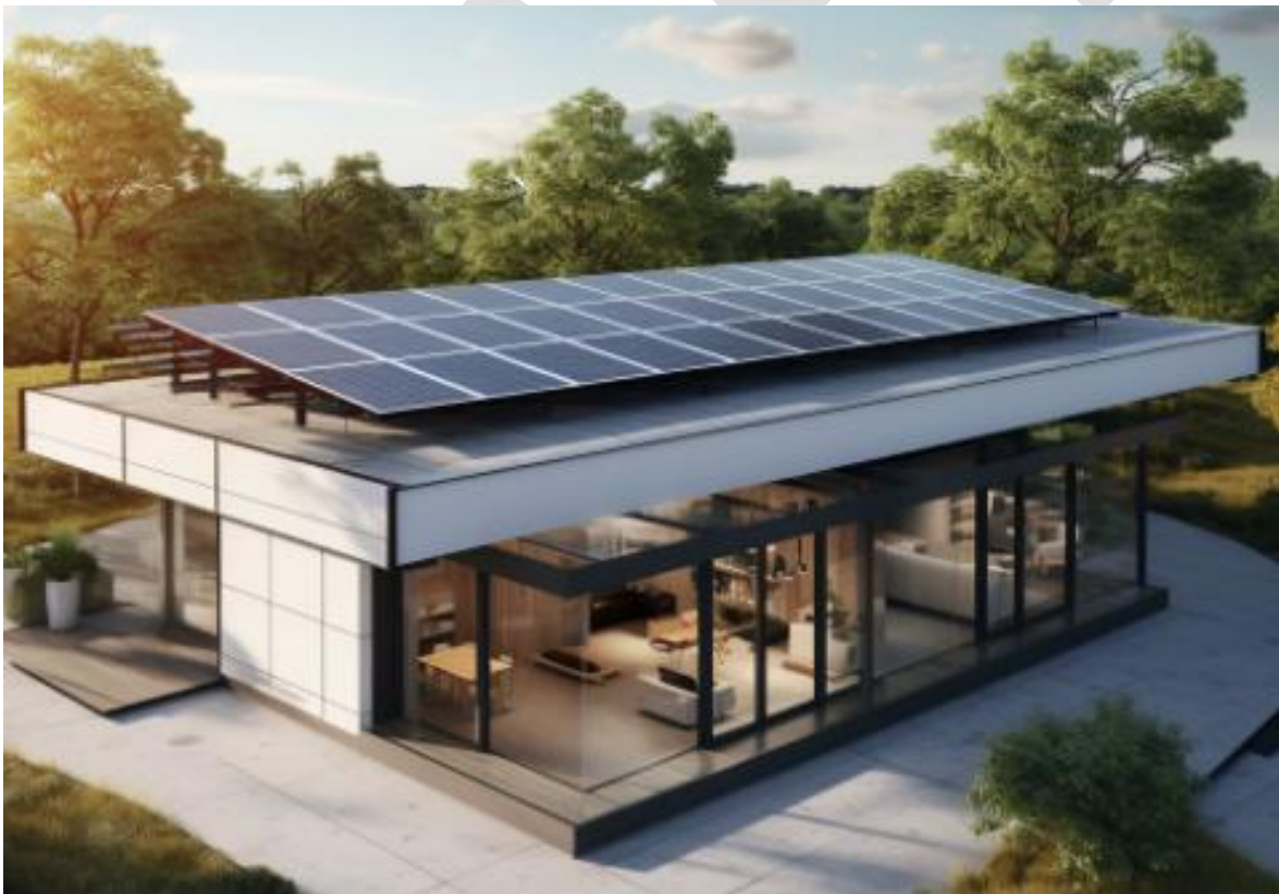
Panels on a flat roof without a parapet, mounted in an organized pattern aligned with the edges of the roof.
