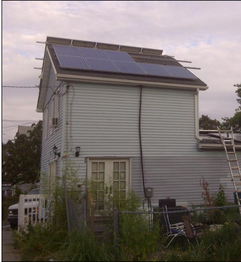
Panel-related equipment extends beyond the roof and is not colored to match the surface to which it is attached.
