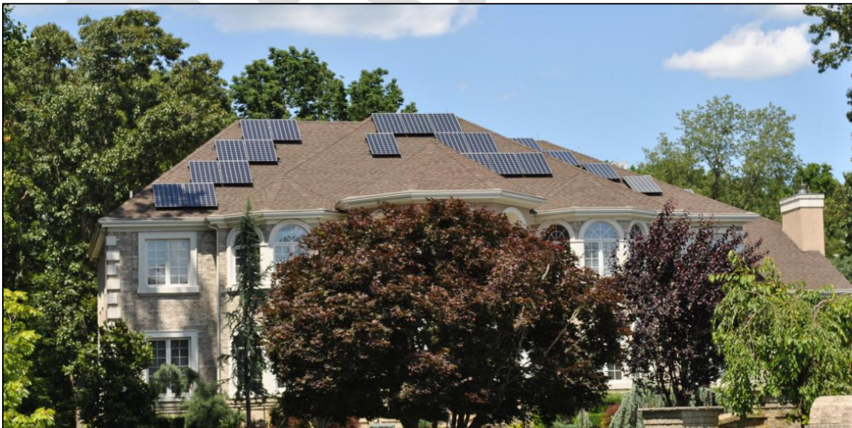
A disjointed arrangement of panels on multiple roofs.
